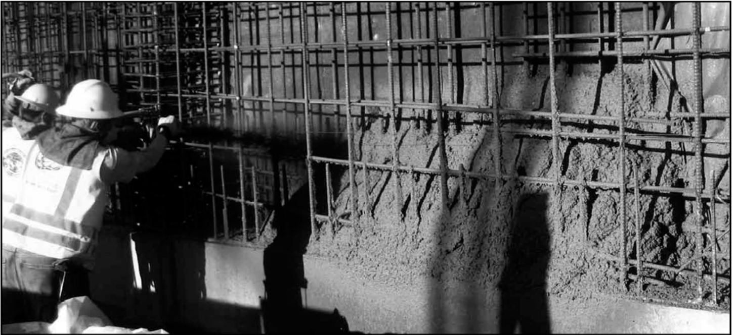
PHOTO 2: SHOTCRETE FOUNDATION WALL
