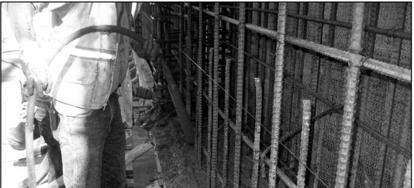
PHOTO 1: KICKER FORM AT BASE OF SHOTCRETE WALL
