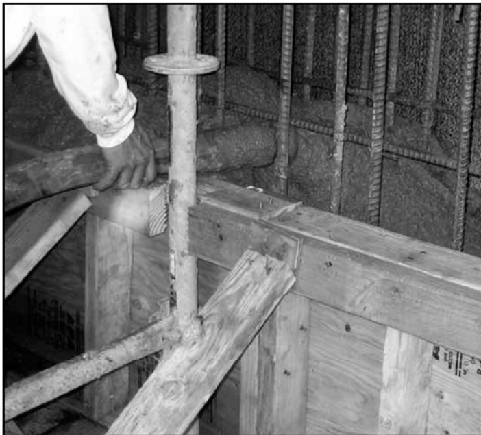
Photo H3-3: SHOTCRETE PLACEMENT IN KICKER FORM
